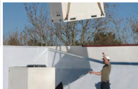
A large crane lifts one of 17 Reznor PreevA units onto the rooftop of the LEED-certified YMCA building.
