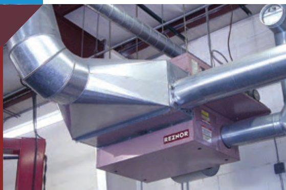
Brian Sinclair, owner of Cummins Automotive, appreciates that his Reznor waste oil heater paid for itself in less than two years. Reznor waste oil heater mounted in ceiling at Cummins Automotive Garage.
