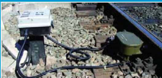
PMA's polyamide cable protection is used for rail infrastructure to protect against rocks and gravel.
