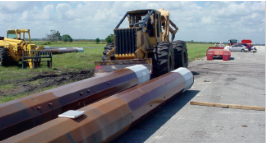
T&B fabricated and shipped poles to Florida to support reconstruction efforts.
