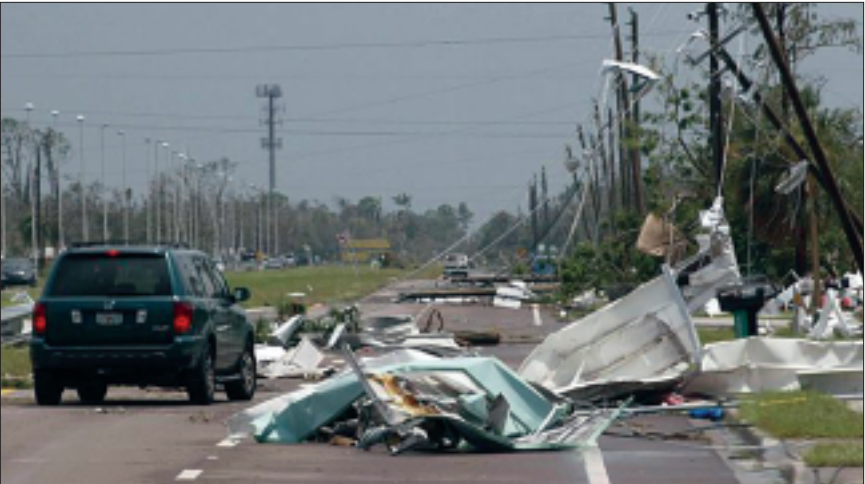
Hurricanes downed power poles and lines throughout Florida.
